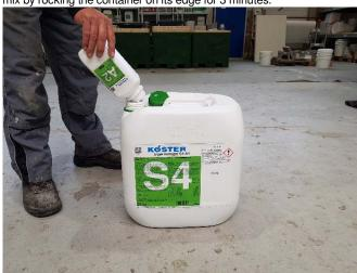
For the standard mixture, which gives a gel time of 40 seconds at 70°F, pour the entire B-component into the empty canister and fill with 20 kg of water to a height of 8.25 inches (can be marked in advance), seal, and mix by rocking for 30 seconds. The green canister can be cleaned and re-used.
